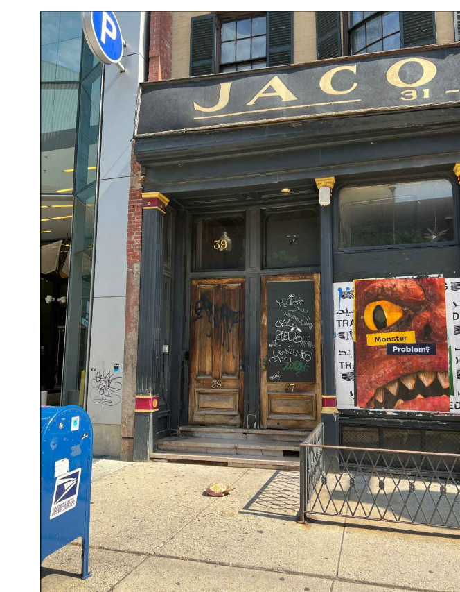
PHOTOGRAPH - EXISTING FRONT LEFT ENTRYWAYS
